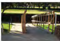
Temporary Route During Construction
